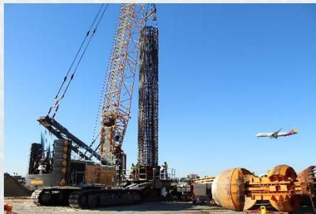
Once the pile has been excavated to depth, a reinforcement cage is installed and concrete is placed directly into the drilled hole while the casing is simultaneously removed.
