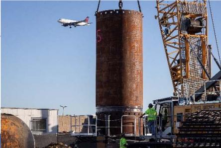
Cast-In-Drilled-Hole (CIDH) piles are commonly used in the construction of bridge structures, and refer to a construction method in which the reinforced concrete piles are cast in drilled holes to predetermined elevations using a heavy wall steel casing to prevent caving. CIDH methodology varies based on several factors, including soil composition, the presence of groundwater and construction impact considerations.
