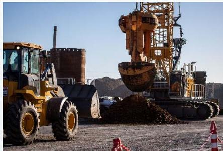
In order to mitigate dust, vibration and sound impacts due to construction, LINXS will use the oscillator method for large diameter CIDH pile construction, advancing the casing into the ground (without the use of impact or vibratory hammers) while concurrently excavating the displaced soil and rock. The drilling casing preserves the integrity of the drill hole, even in unstable or wet ground formations.
