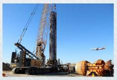
Once the pile has been excavated to depth, a reinforcement cage is installed and concrete is placed directly into the drilled hole while the casing is simultaneously removed.
