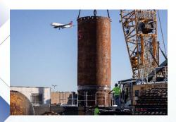
Cast-In-Drilled-Hole (CIDH) piles are commonly used in the construction of bridge structures, and refer to a construction method in which the reinforced concrete piles are cast in drilled holes to predetermined elevations using a heavy wall steel casing to prevent caving. CIDH methodology varies based on several factors, including soil composition, the presence of groundwater and construction impact considerations.
